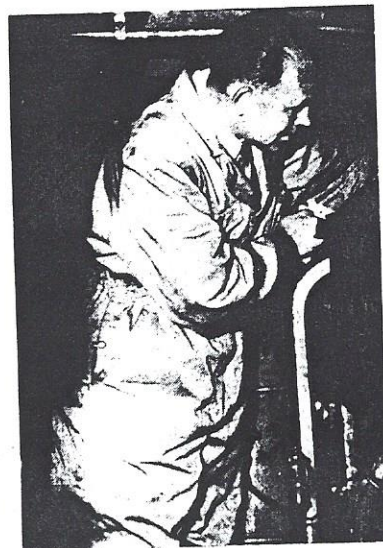
Engine compartment has ample working space. Motive power is supplied by 1200 h.p. diesel. The locomotive pulls ten coaches. The train was designed only for coach service, has top speed of 102 m.p.h.
